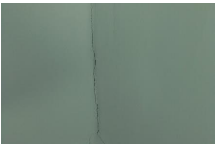
Pic 4 – Crack on wall
